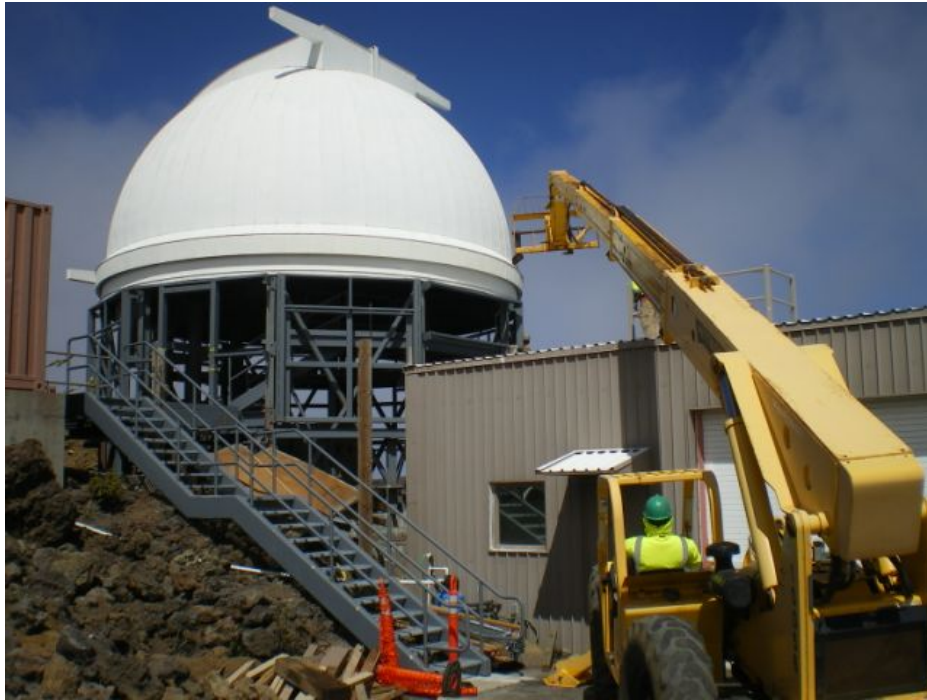
Figure 2. The new stairway from the PS2 catwalk to the Pan-STARRS driveway.
